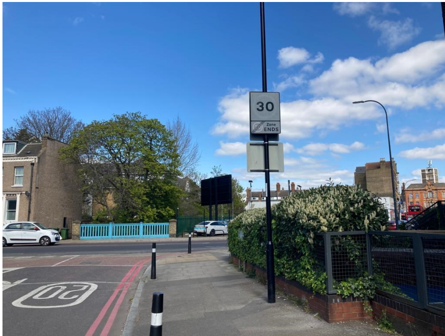
Bridge over River Quaggy from Brightfield Road
