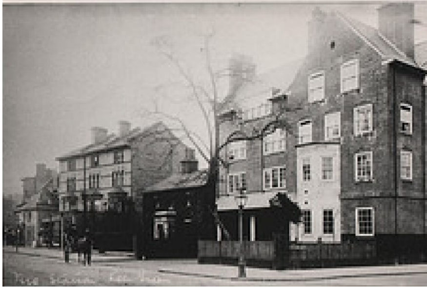
Lee Green Fire Station
