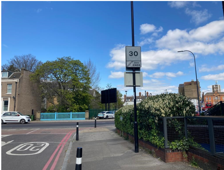
Bridge over River Quaggy from Brightfield Road
